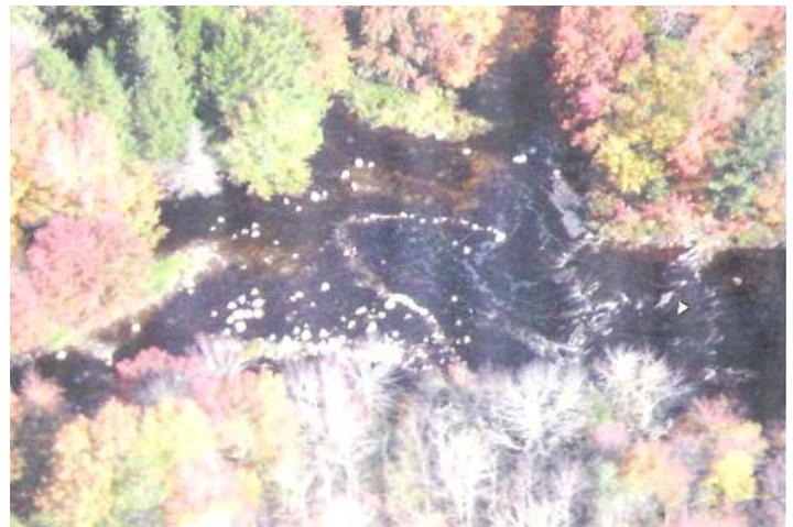
Aerial view of the Roderick Ford stone weir (BcDh-26)
